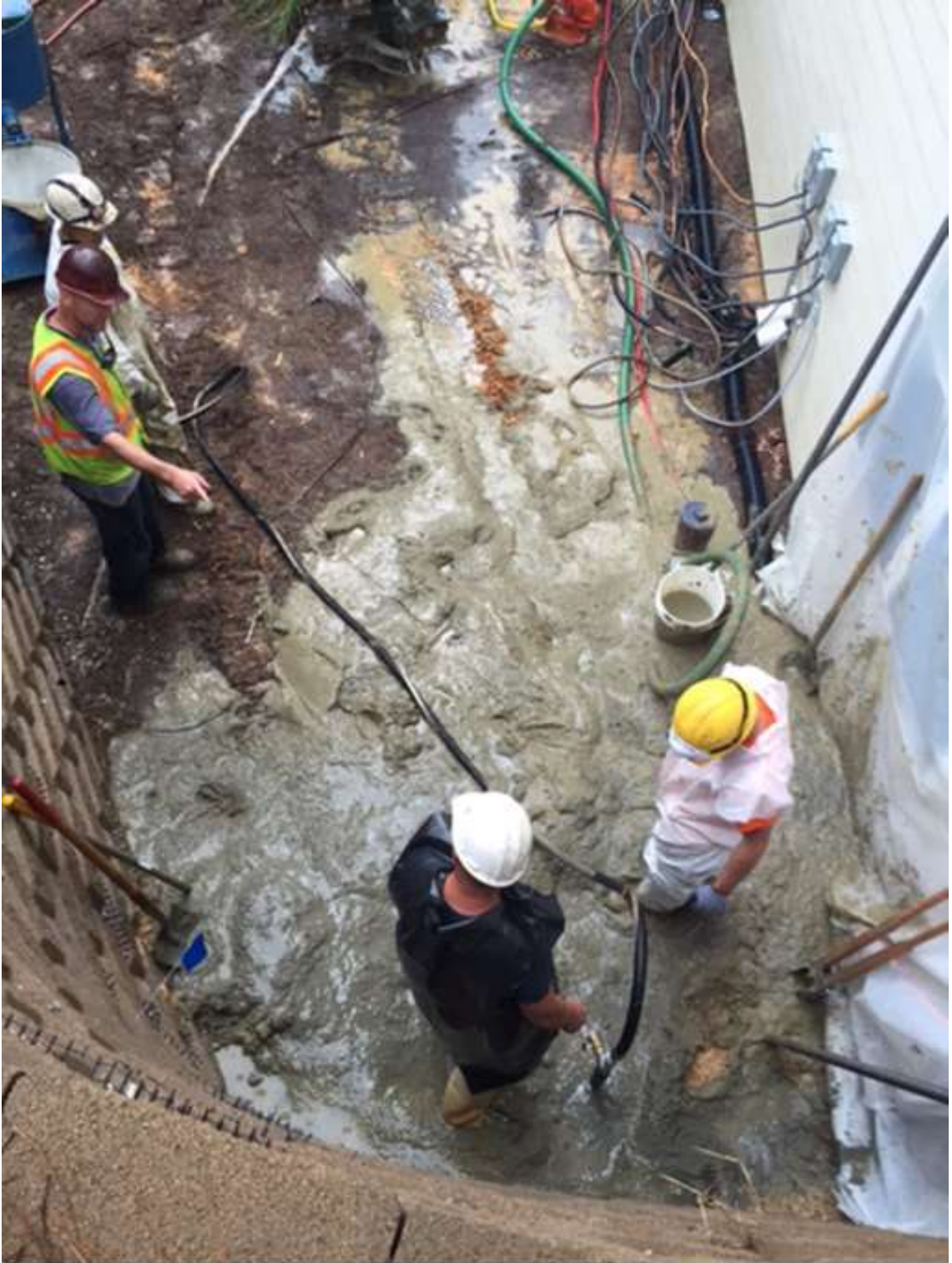
Figure 3. Pumping grout from the center bar of the installed pile.
